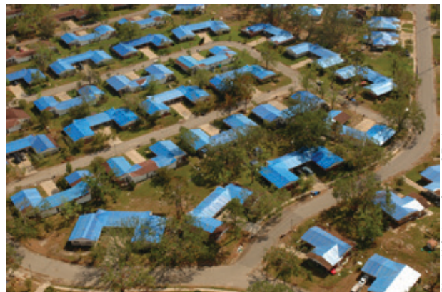
Photo: U.S. Army Corps of Engineers
